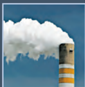
AIR POLLUTION CONTROL
