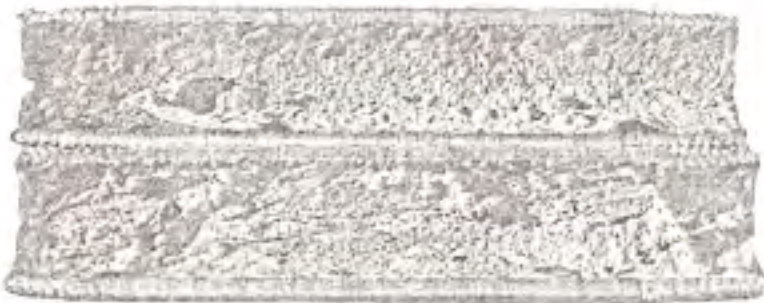
5. Specimen removed from old pipping from new water heater six months after installation of electrostatic descaler..
